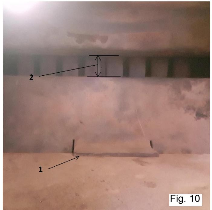
Fig 10 shows the baffle position as viewed from inside the firebox. Item 1 on the picture highlights that the tab on the baffle must overlap down over the vermiculite lining at the rear of the firebox. Item 2 shows the gap to the front between the baffle and the body of the appliance, this should be approx 20mm
